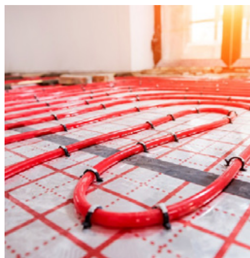
UNDERFLOOR HEATING SYSTEM
